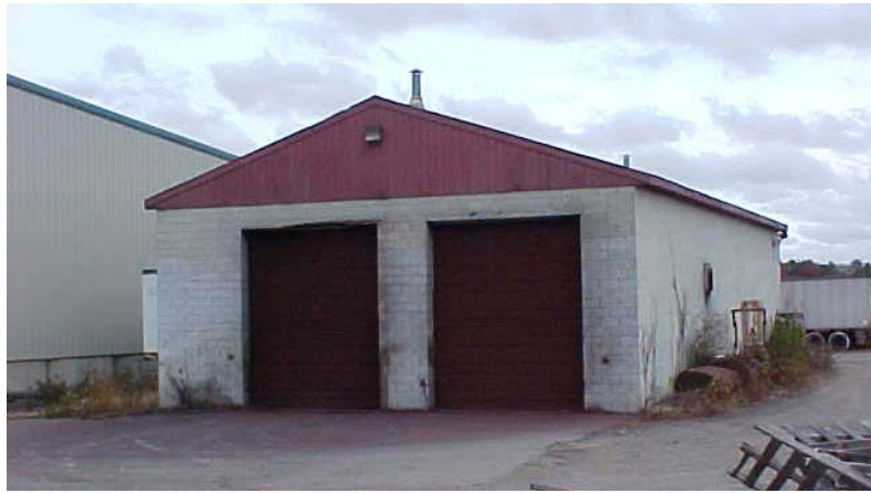
Building 1 - Rear View
