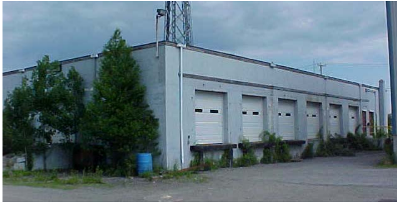
Building 2 - Rear View
