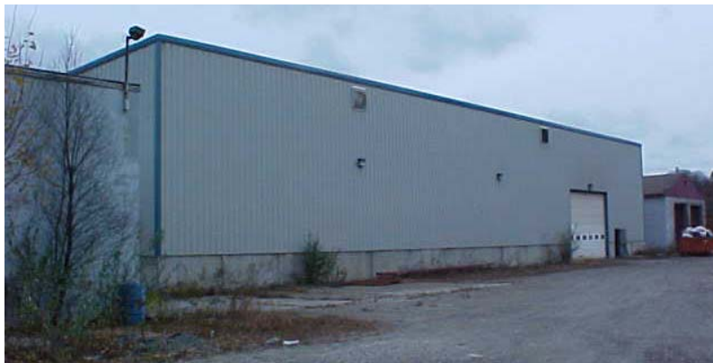
Building 3 - Rear View
